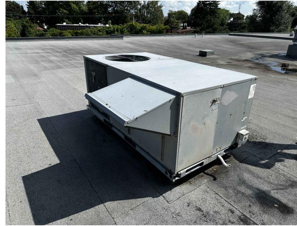
PHOTO 1: UNITÉ DE VENTILATION UTA-3 À DÉMOLIR ET REMPLACER
